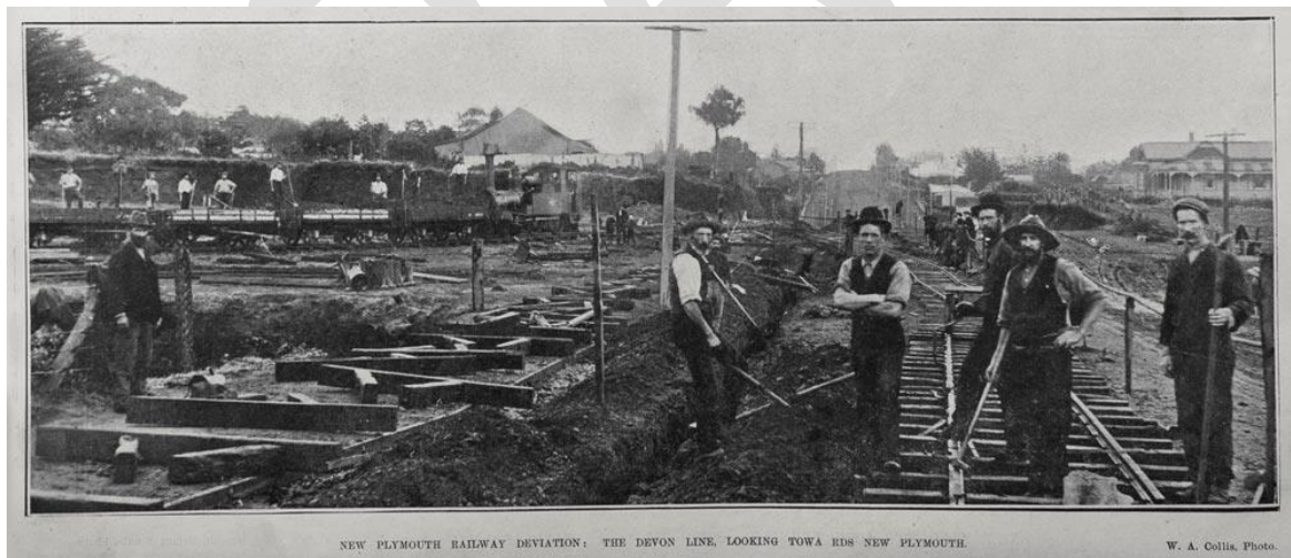
Devon Street East looking west towards New Plymouth from about present site of The Federal Store café. These railway tracks were temporary arrangements to facilitate construction. Auckland Weekly News , 9 August 1906, page 6, Sir George Grey Special Collections, Auckland Libraries, AWNS-19060809-6-5.
